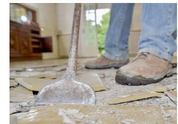
Vinyl sheet flooring, floor levelling compound, floor tiles
