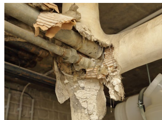
Pipe and duct coverings
