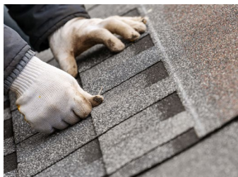
Built up roofing and felts, roof shingles/siding
