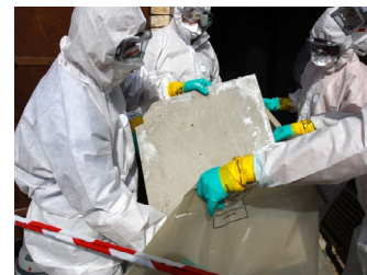
Drywall and cement sheets
